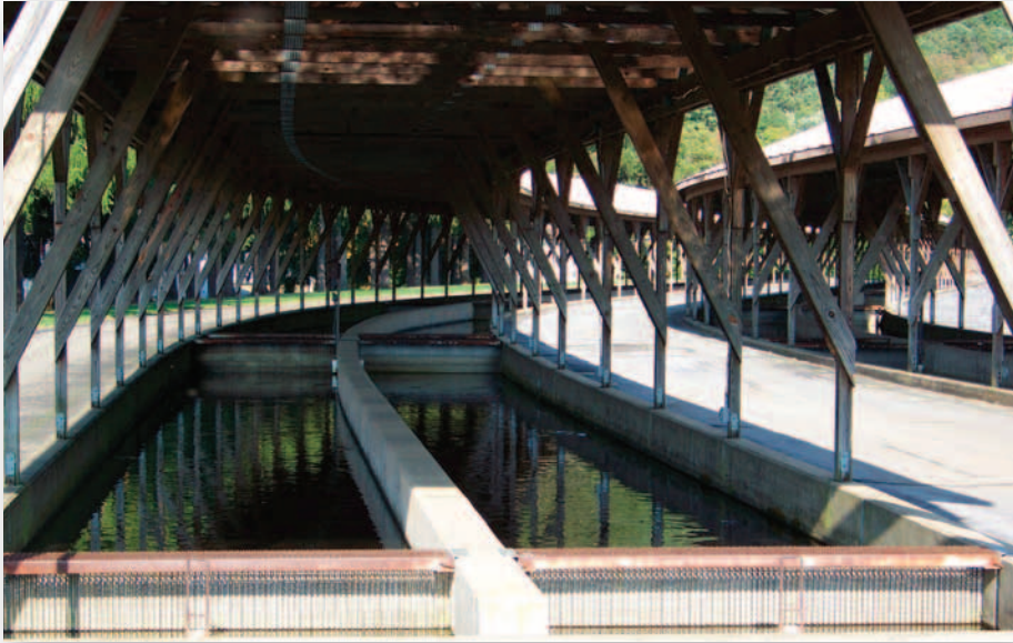
There is a series of 40 raceways at Tionesta State Fish Hatchery used to rear steelhead fingerlings.
