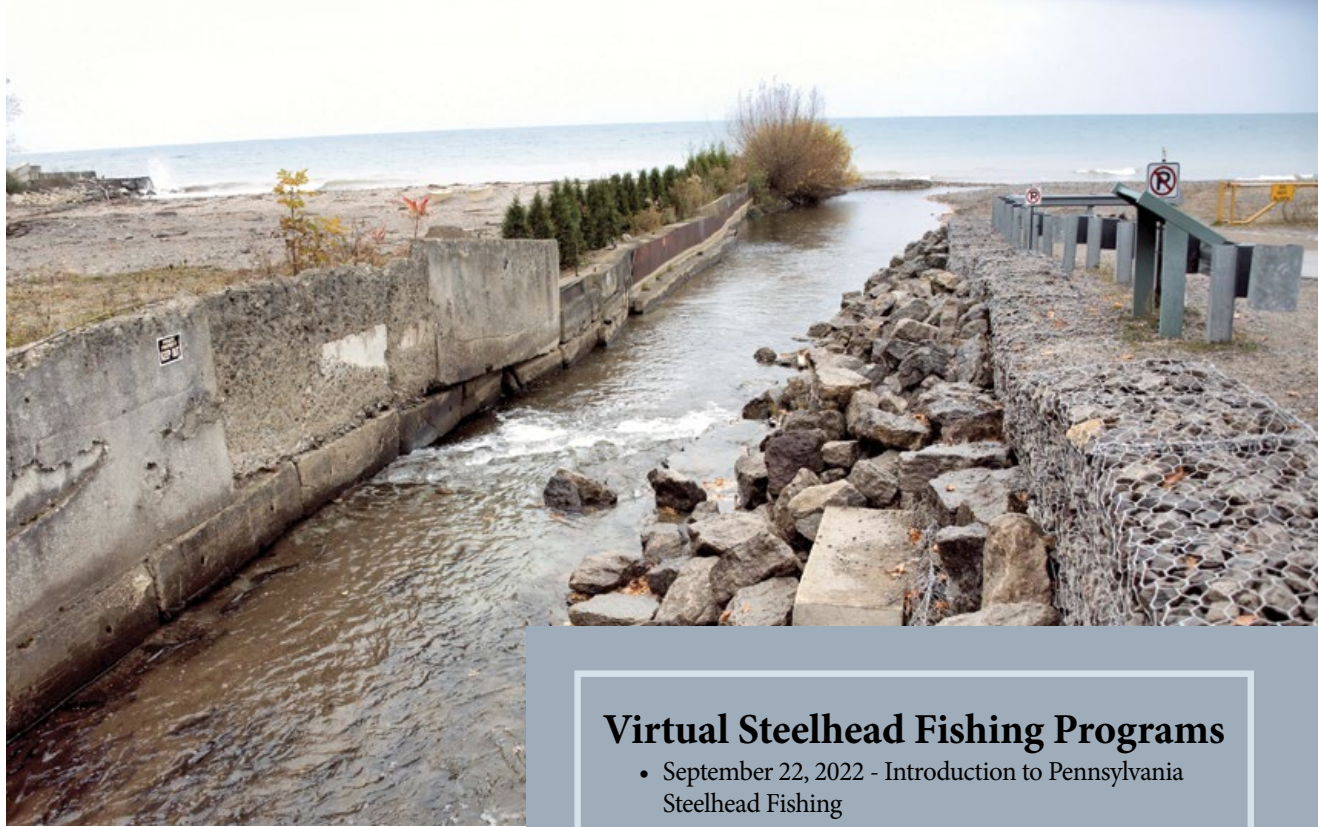
The walls at the bottom of Trout Run create a long narrow trough that ends with a gate several hundred feet upstream as it empties into the lake.
