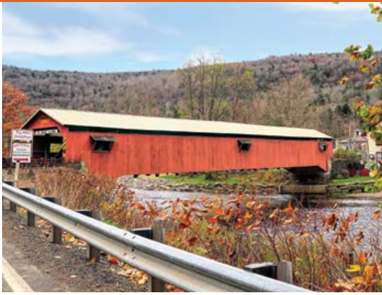
Forksville covered bridge
