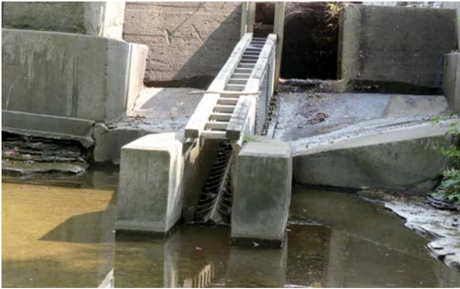
The PFBC used grant money to build a 30-foot aluminum fish ladder.
