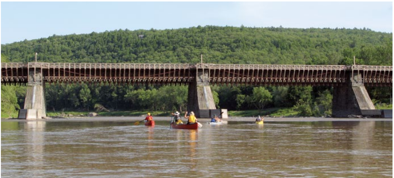
Paddlers on the Delaware River Sojourn prepare to head under the historic Roebling Bridge near Lackawaxen, PA—the oldest existing wire suspension bridge in the United States. Originally, this bridge carried barges on the Delaware and Hudson Canal over the river in an aqueduct.
