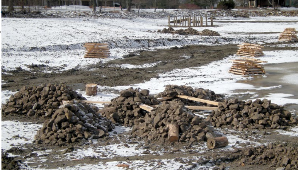
Spider-hump structures combine rock-rubble humps and wood connectors. This photograph was taken when the habitat improvements were nearly completed.
