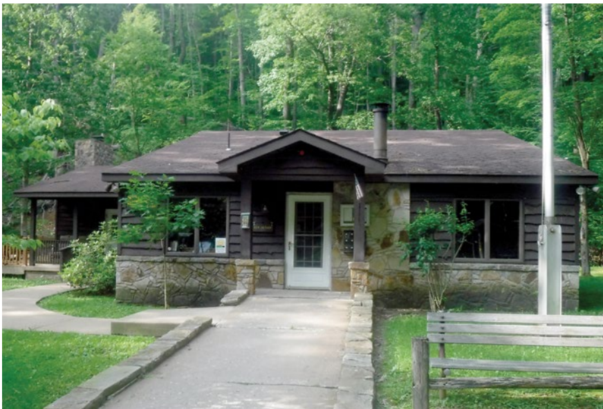
The park office at Linn Run State Park, Westmoreland County, is centrally located.
