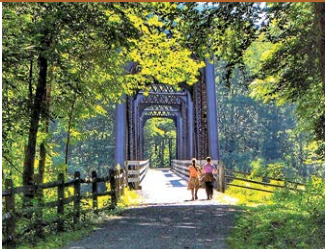
The Cedar Run steel truss railroad bridge provides a stunning landmark on the Pine Creek Rail Trail.
