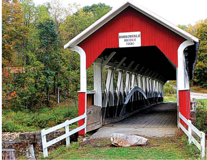
Barronvale Bridge, Somerset County
